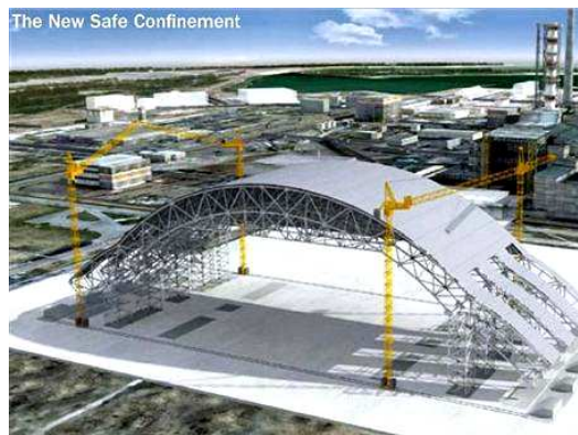
The New Safe Confinement
